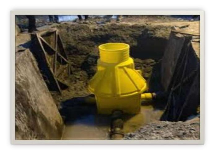
In areas where the soil is very loose and we are encountered with landfills, it is recommended to remove an amount of soil from the floor and replace it with suitable soil, and then the abovementioned steps are performed. These cases must be done by engineers and consultants opinions. Since the transferring of dead and live and also pressing forces are dragged down at the base of manhole, the equipments
